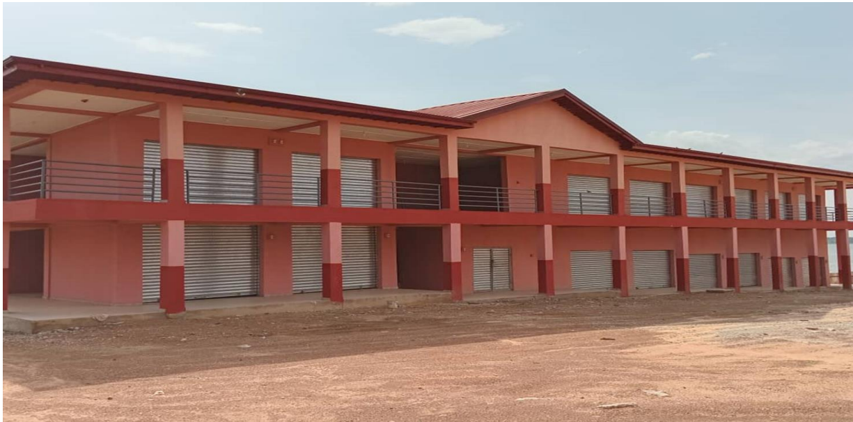
CONSTRUCTION OF 32-UNIT LOCKABLE STORES AT DAMBAI MARKET
